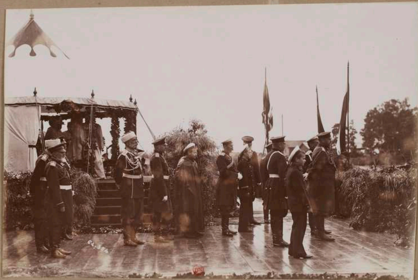
Construction of a military port in presence of S. M. the Emperor
